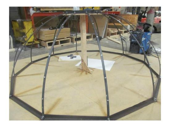
Bolt together the base ring. Parts bolt together with matching lettered parts. The base comes in two pieces. Bolt the ends pieces together to hold base while placing longitudinal ribs on.
